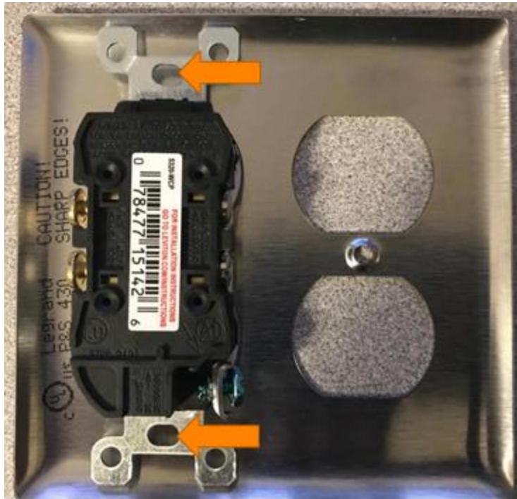
Figure 3-5 – Marking the mounting holes in the stainless-steel faceplate
