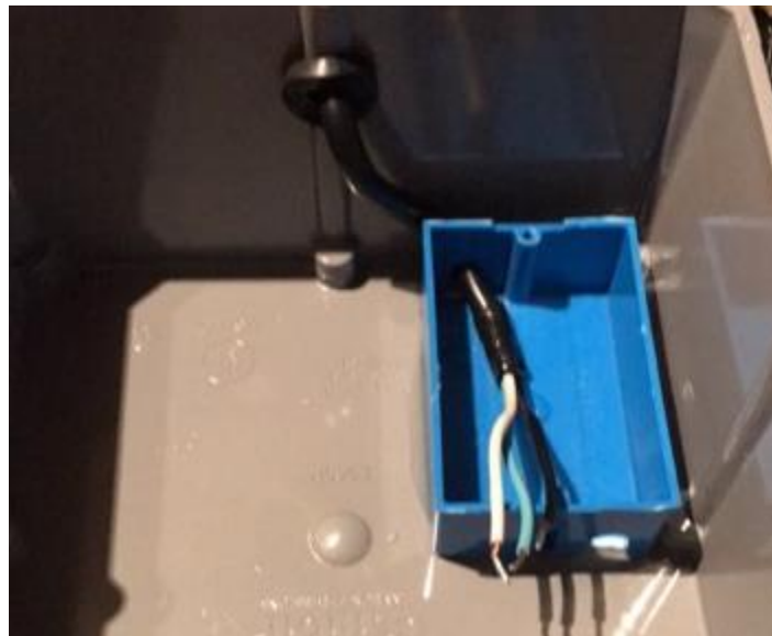
Figure 3-1 – Pull Through the Main Power Supply Cable
