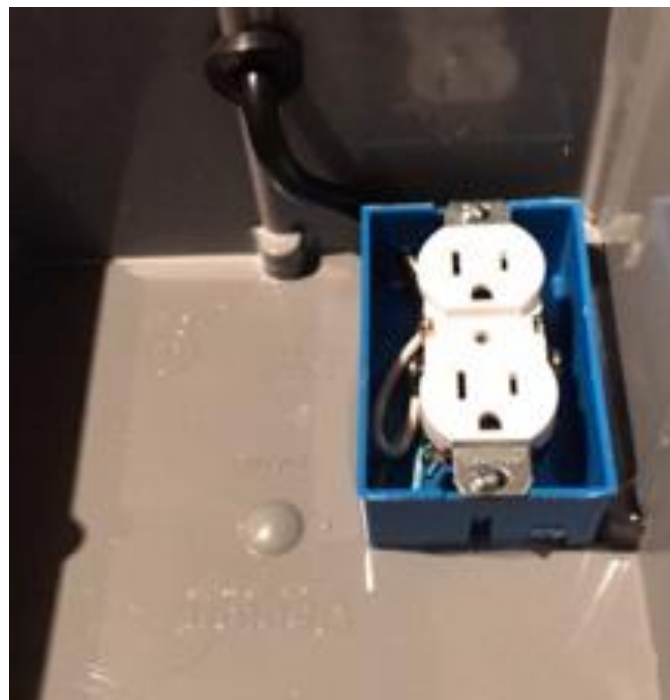
Figure 3-3 – Completed Internal Power Supply Wiring
